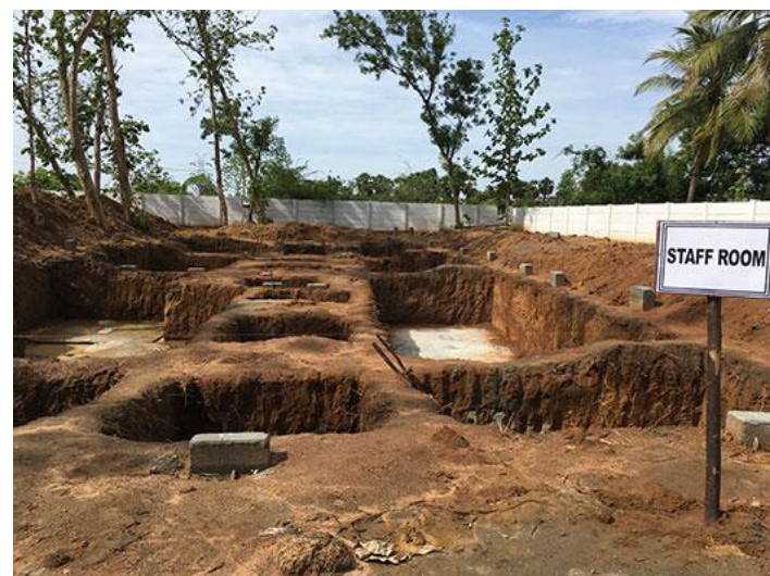
Start of marking and excavation
