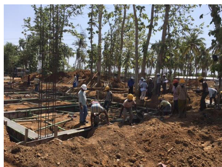
Casting of plinth beams: Staff Room
