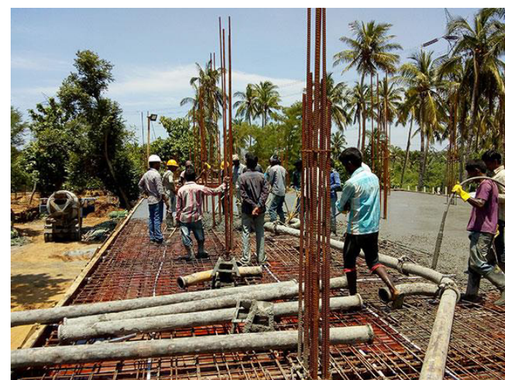
Preparing to cast roof slab
